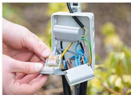
Connecting a bollard light
