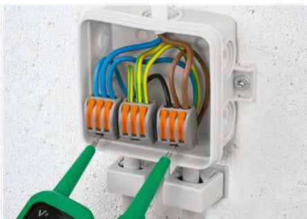
Testing the wired connectors.
