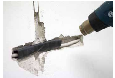
Heat the shrink tube and properly reclose the damaged area.
